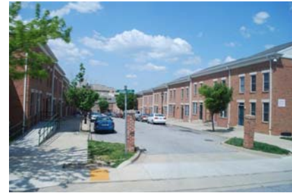
Mixed-income housing at Pleasant View Gardens, a HOPE VI site included on the tour
